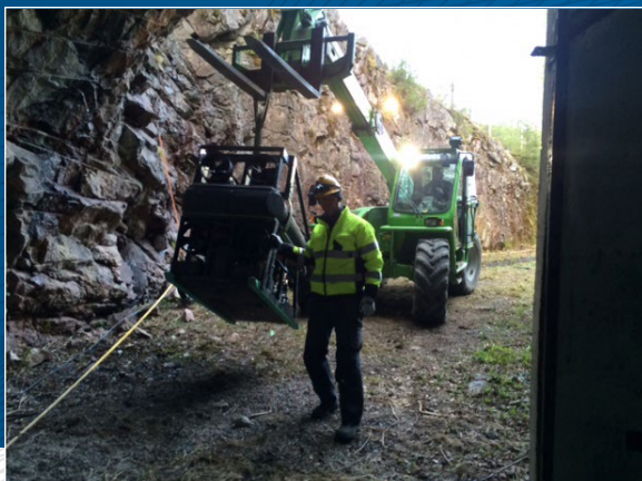
The ROV is driven down access shaft to the entry point of flooded tunnel
